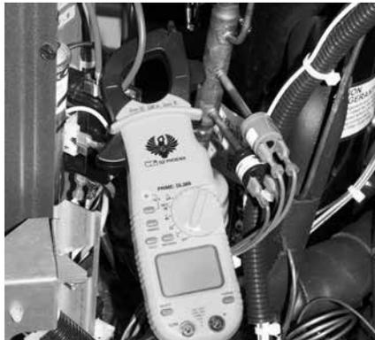
If there is no change in amps, then the compressor is not shifting.
